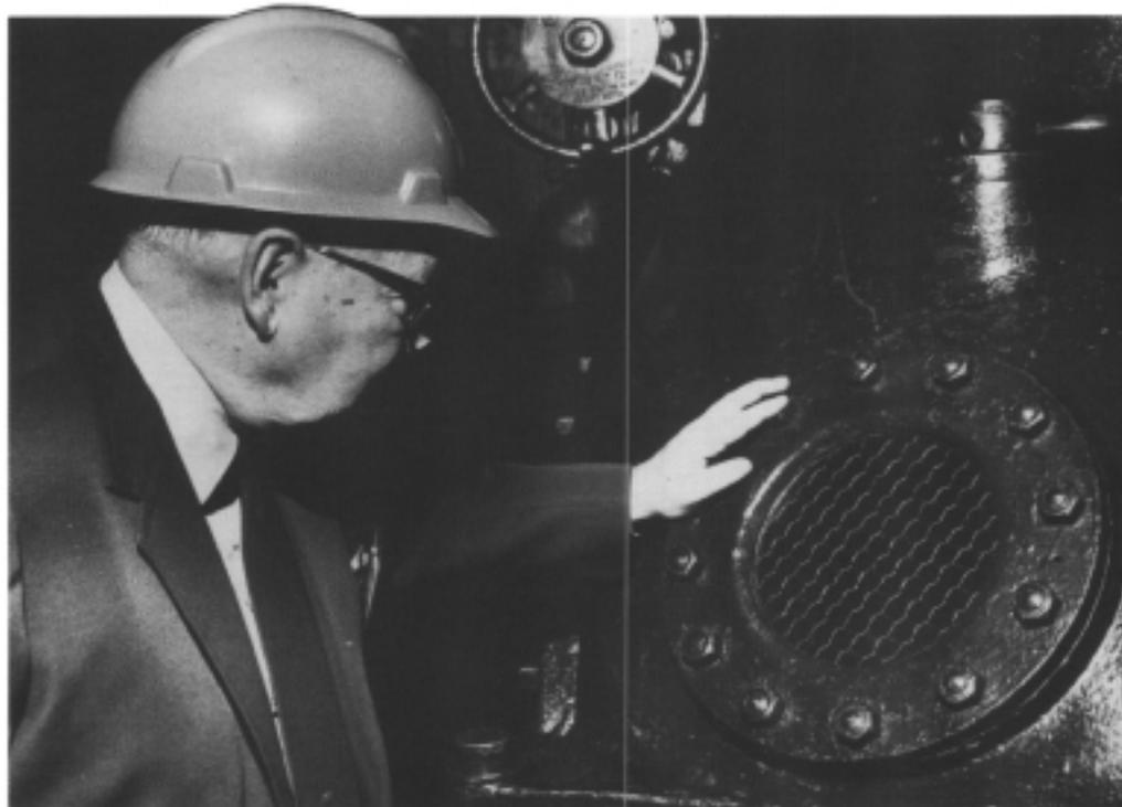
*Former Holtwood superintendent W. Roger Small Jr. checks the glass inspection port on the Unit 5 thrust deck that enables operators to view the oil-bathed bearing during operation.*
