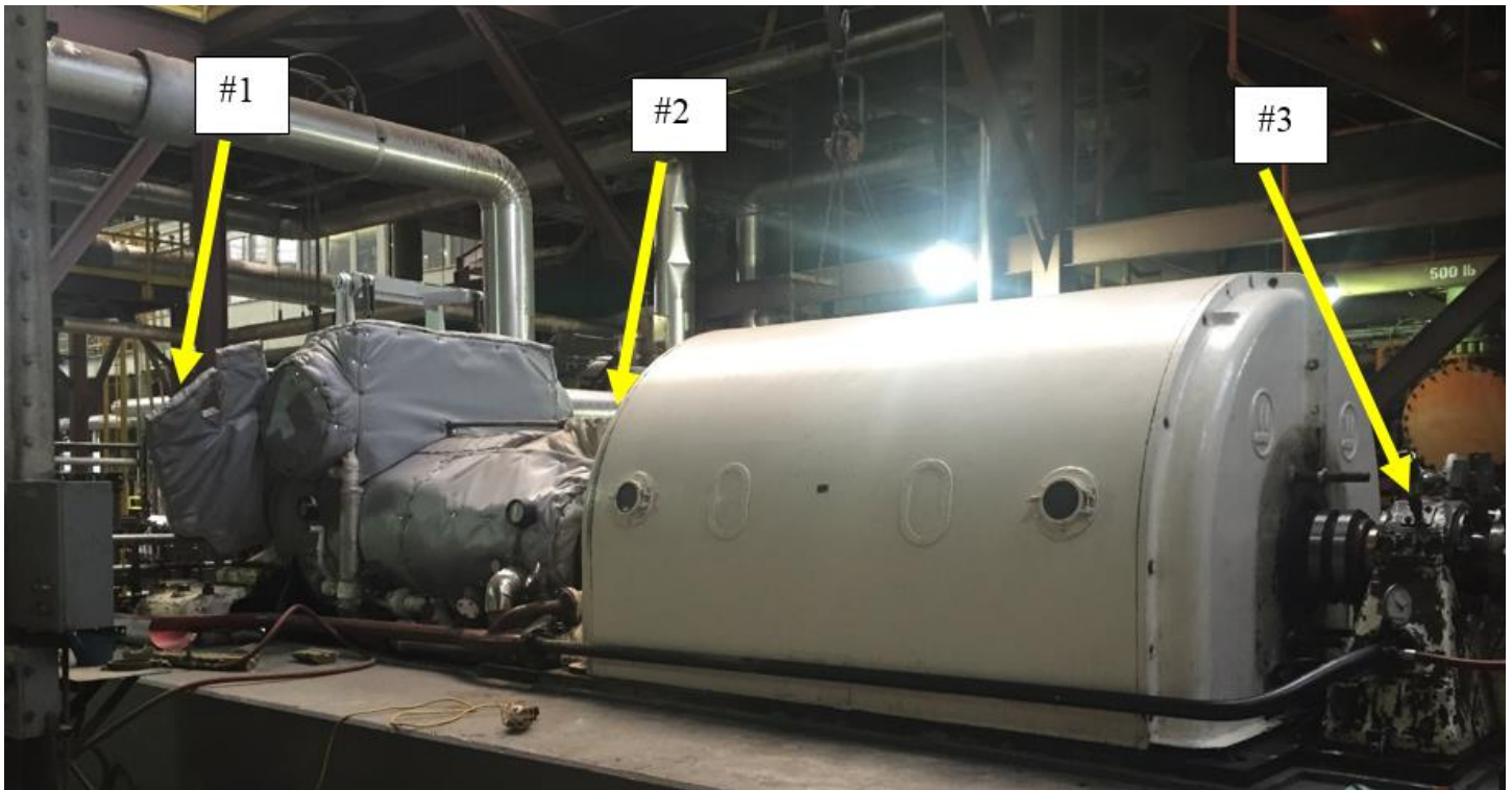
Figure 10 - Turbine Generator Balance/Measurement Planes
